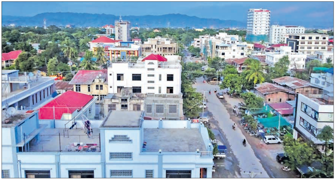
Experts need to assess risk for buildings in Mandalay City. PHOTO: MAUNG PYI THU
