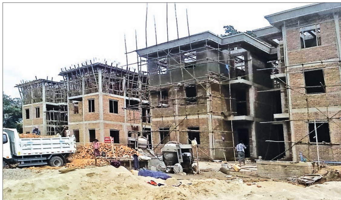
Buildings under construction for accommodation of service personnel in Natogyi Township.
