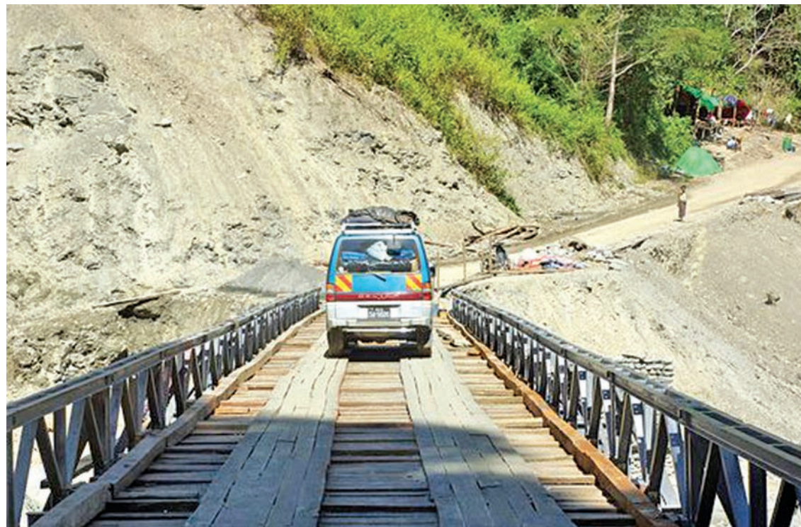
A new bailey bridge lies on Chichaung Creek in Mindat Township. PHOTO: DISTRICT IPRD
