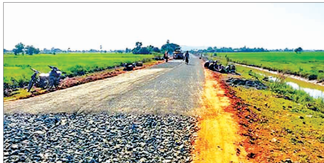
Construction of Kyunhla-Chatthin-Kawlin road in progress. PHOTO: KO KO MAUNG (KAWLIN)
