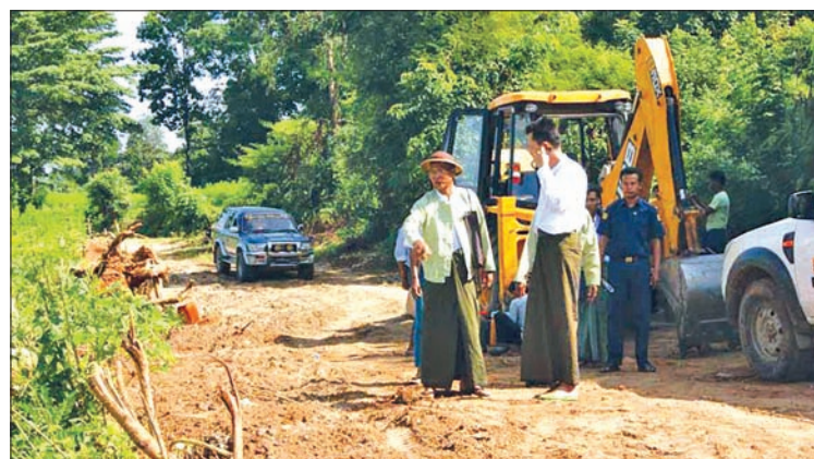
Officials inspect progress of earthen road. PHOTO: THAN HTAY AUNG
