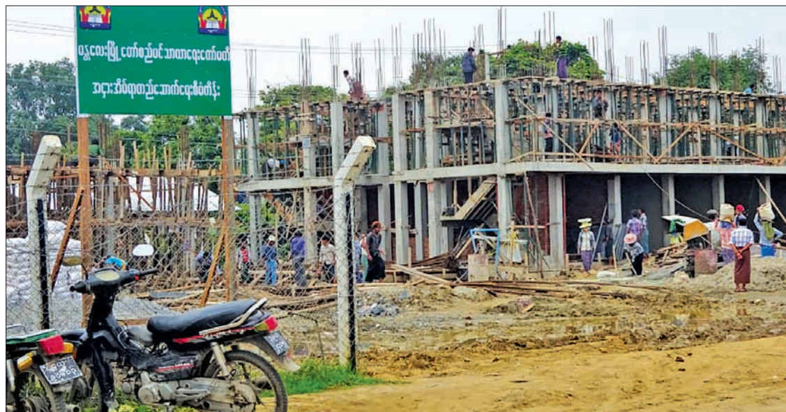
Apartments under construction for homeless in Mandalay Region. PHOTO: MAUNG PYITHU
