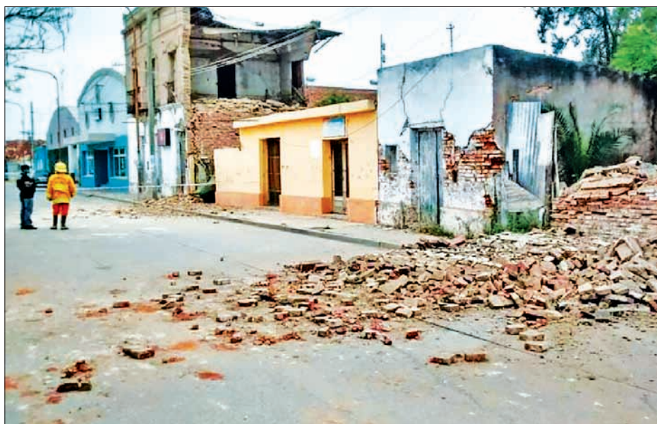
Debris of a wall are seen in street after an earthquake in El Galpon locality, Salta province, Argentina, on 17 October, 2015. PHOTO: XINHUA
