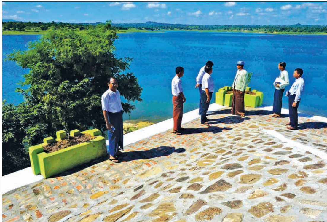
Local authorities inspect maintenance of Sintaewa Dam. PHOTO: U ZAW MIN NAING
