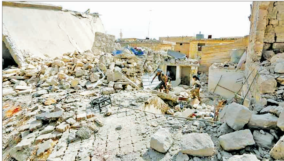
Residents inspect a site hit by what residents said were airstrikes carried out by the Russian air force in the town of Darat Izza in Aleppo's countryside, on 13 October 2015. PHOTO: REUTERS
