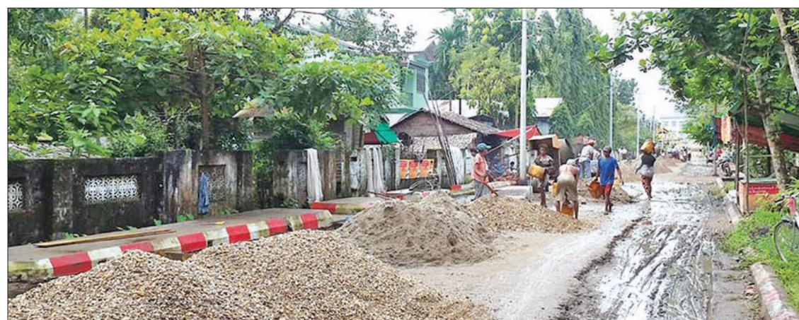
The 1,100-foot long asphalt road stretching in Nyaungdon. PHOTO: TUN KYAW
