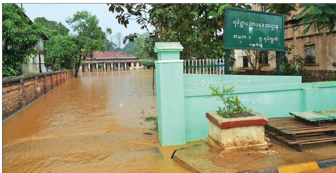
Floodwater enters school compound in Kyaukme. PHOTO: U MYINT AUNG
