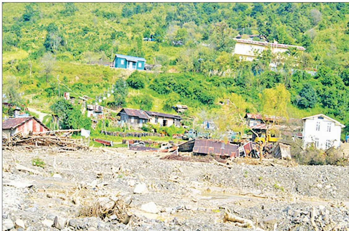
Homes destroyed by landslides in Haka due to torrential rain in July. PHOTO: MNA
