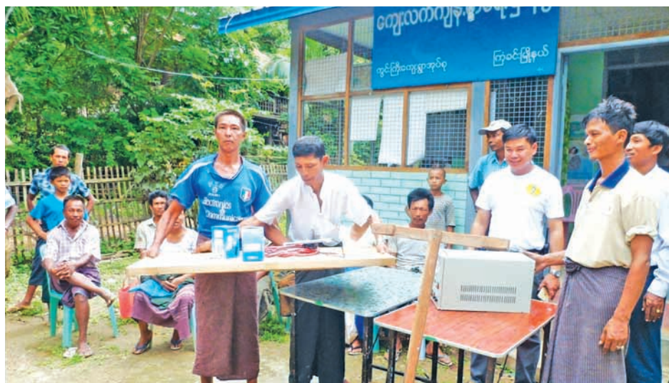
Kwingyi villagers prepare to install solar panels. PHOTO: DRD
