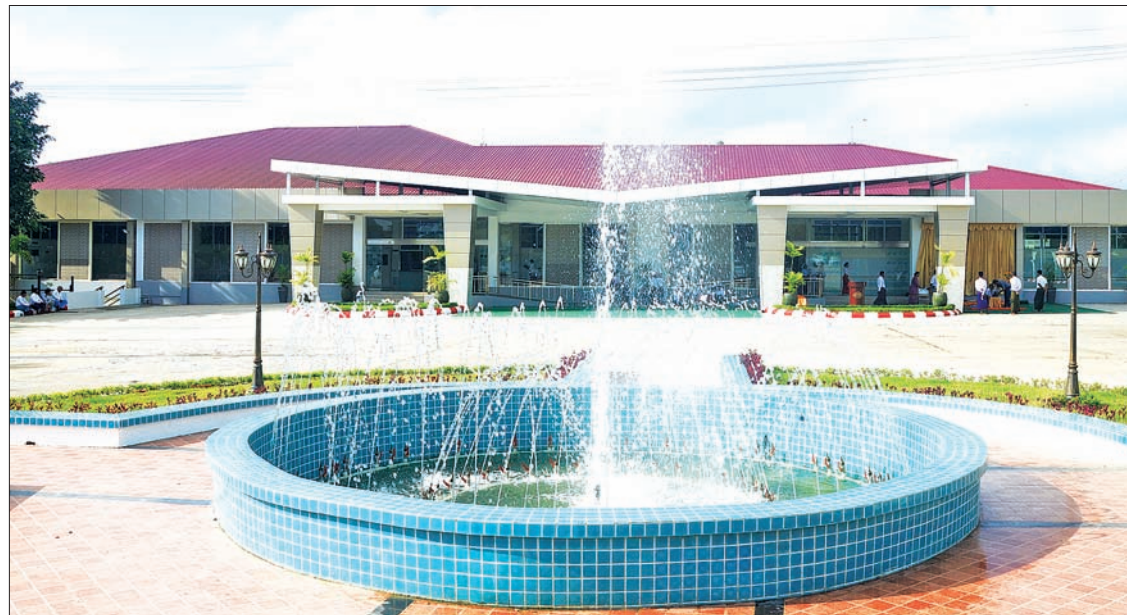
Construction of the hospital began in December 2013 and it cost approximately US$1.7 million. PHOTO: MNA
