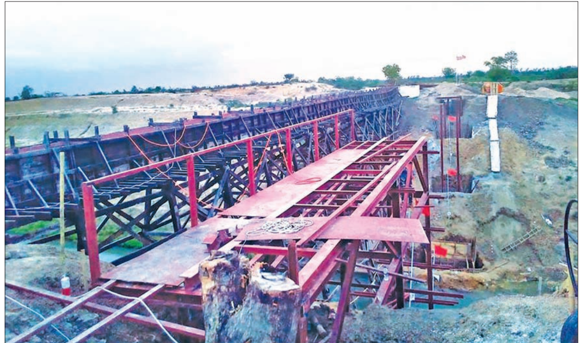
Irrigation Department installs steel gutter crossing new tributary in Linzin irrigated area in Salin Township.—PAING ZAY-MAGWAY
