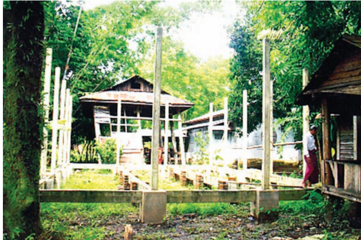
Kaylartha Golden Monastery under construction in Nyaunglaybin Township.—NAY LIN (NYAUNGLAYBIN)
