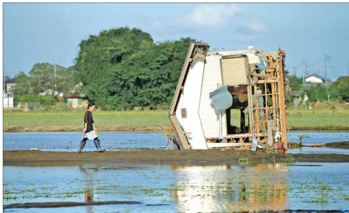
A woman walks towards a collapsed house on a field inundated by floodwaters in Joso in Ibaraki prefecture on September 11, 2015. Thousands of rescuers arrived in a deluged city north of Tokyo on September 11 to help evacuate hundreds of trapped residents and search for 12 people missing after torrential rains triggered massive flooding.—AFP
