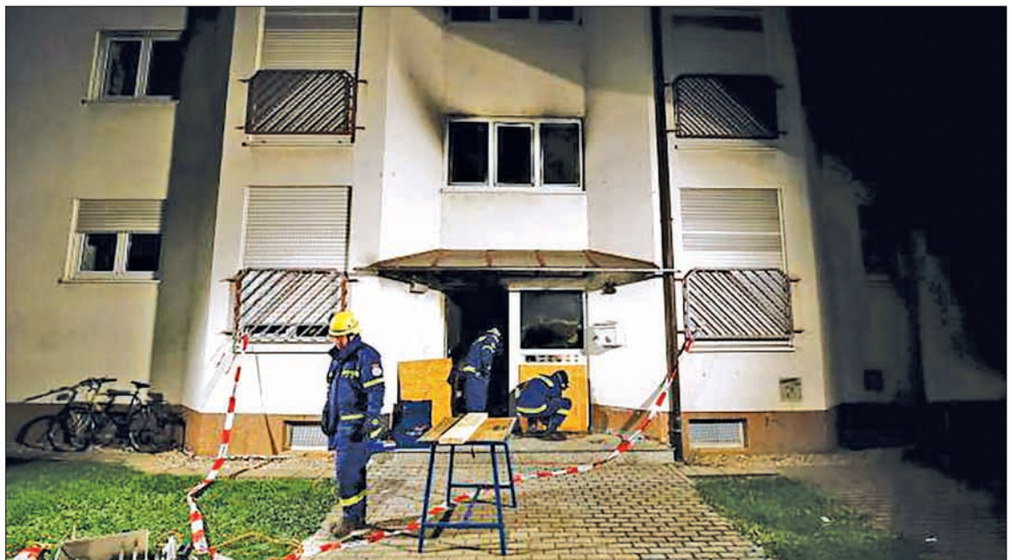
Members of Germany’s technical support unit (THW) fix wooden boards to a building used to house asylum seekers after a fire broke out in the entrance area of the building in Heppenheim, 30km south of Frankfurt, Germany, early morning September 4, 2015.—REUTERS
