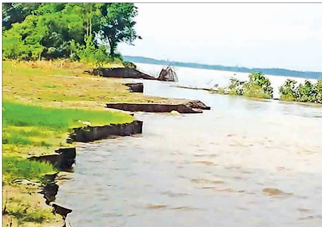
Ayeyawady River eroding bank in Kyangin Township.— Win Bo (Township IPRD)
