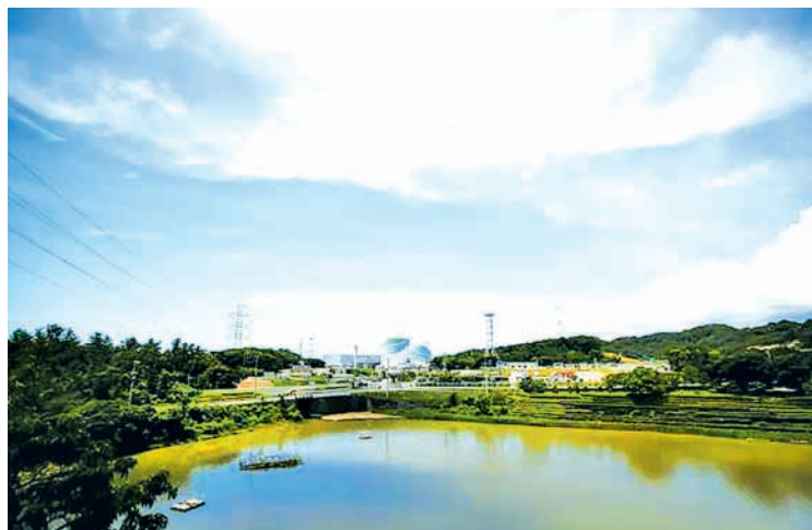
No.1 (L) and No.2 reactor buildings are pictured at Kyushu Electric Power's Sendai nuclear power station in Satsumasendai, Kagoshima prefecture, Japan, July 8, 2015.—REUTERS
