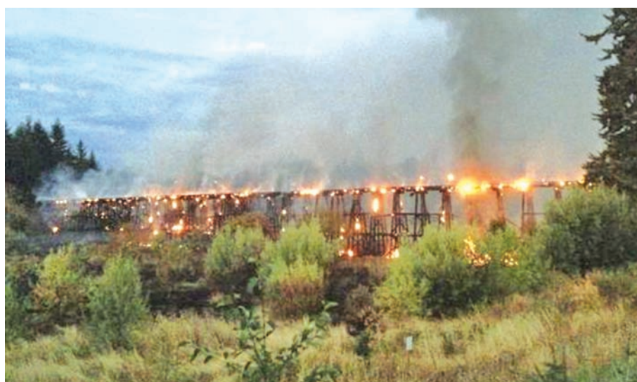
A historic Portland and Western Railroad trestle is seen on fire near Sherwood, Oregon, in this handout photo from the Tualatin Valley Fire and Rescue Department released to Reuters August 11, 2015. REUTERS
