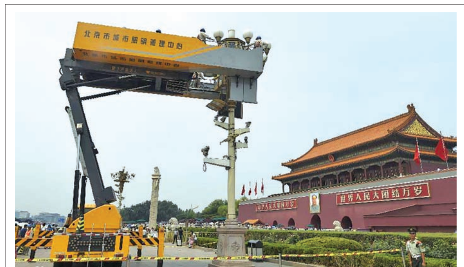
Workers clean and overhaul a lamp during the annual maintenance of city lamps near Tian’anmen Square, in Beijing, capital of China, on 6 July, 2015.—XINHUA
