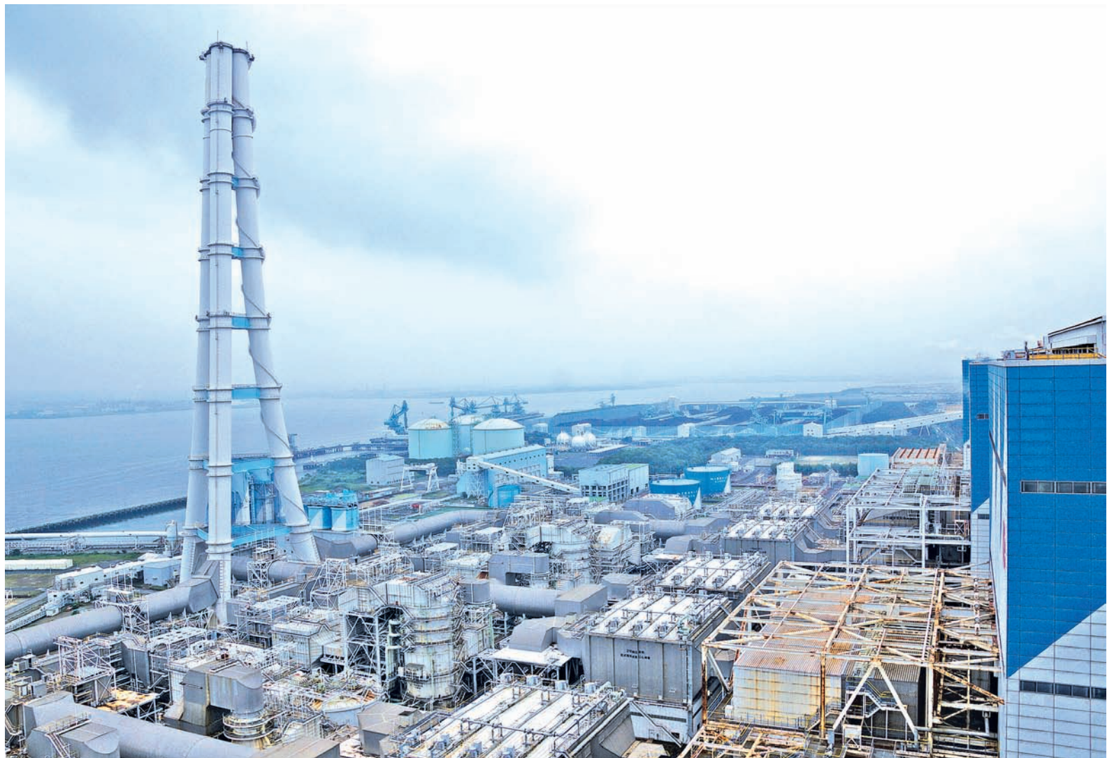
Hekinan coal-fired power plant in Nagoya, Japan.— PHOTO CREDIT: YHT
