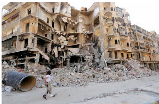
A man walks with the aid of a crutch past damaged buildings in the old city of Aleppo on 27 June, 2015.
