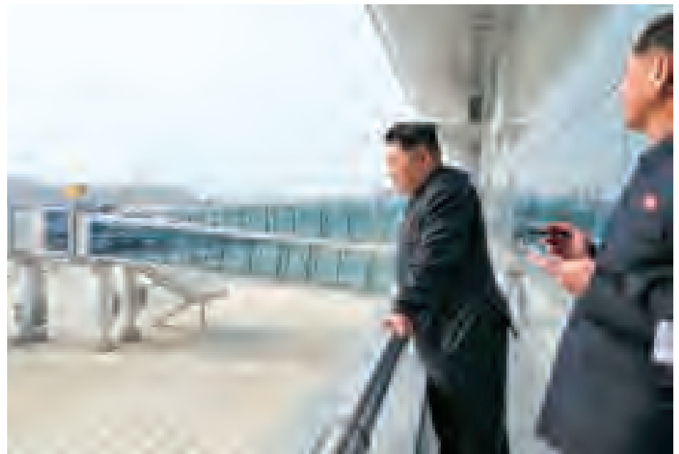
North Korean leader Kim Jong Un (L) gives field guidance at the construction site of Terminal 2 of Pyongyang International Airport, which is nearing completion, in this undated photo released by North Korea's Korean Central News Agency (KCNA) in Pyongyang on 12 April, 2015.—REUTERS
