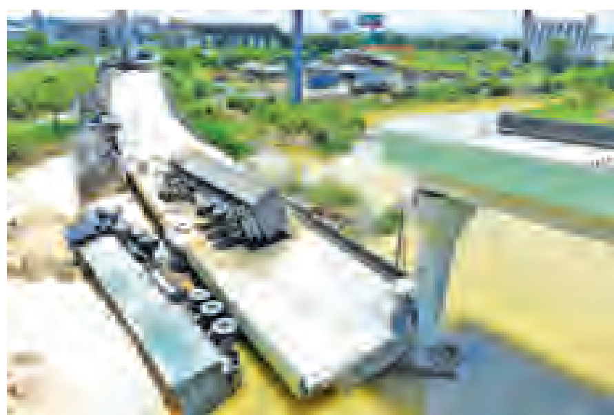
Heavy trucks fall under a highway after a ramp of the Guangdong-Jiangxi Highway collapses in Heyuan, south China's Guangdong Province, on 19 June, 2015. The accident, which killed one person and injured four others, happened at 3:40 am on 19 June (1940 GMT on 18 June) in Heyuan City when a bridge ruptured with four heavy trucks loaded with porcelain clay on it, according to an investigation. The highway, opened to traffic in December of 2005, connects Guangdong with east China's Jiangxi Province.—XINHUA
