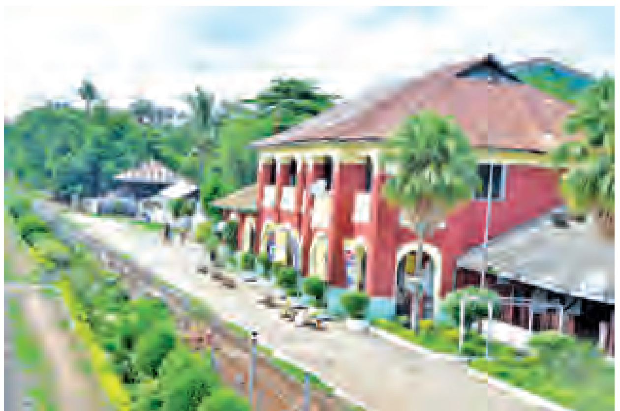
Photo shows Kyimyindine Railway Station with architectural design of colonial era in Kyimyindine Township.
