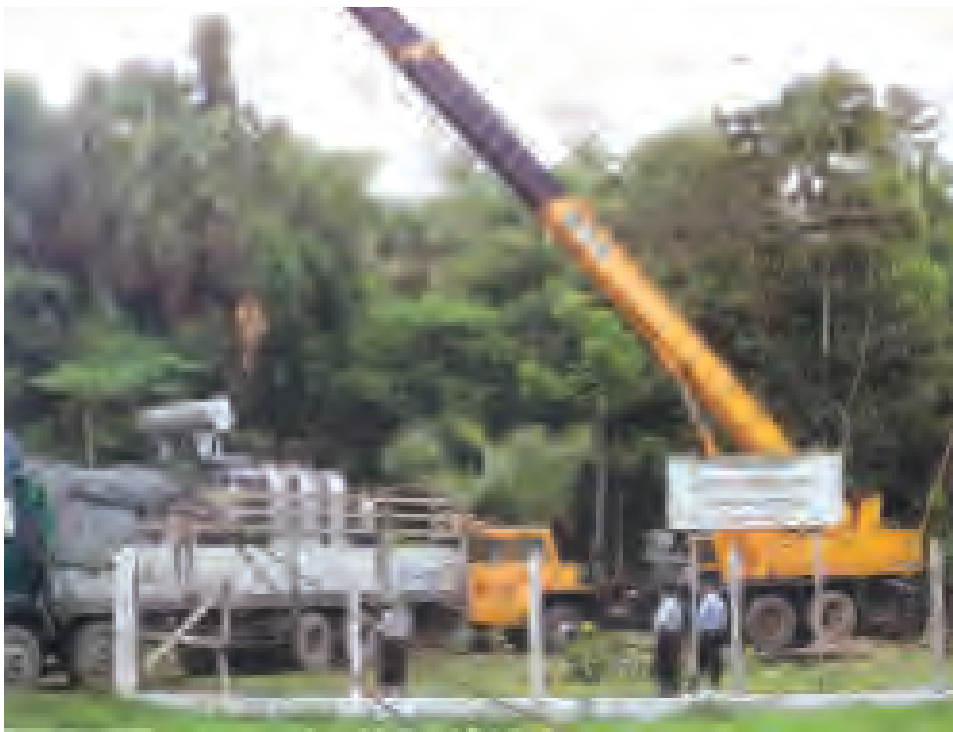
Engineers and skilled workers carry out substitution of 2500-KVA transformer in place of 1250-KVA transformer at sub-power station in Kyaunggon Township, Ayeyawady Region, on 10 June, under supervision of the Patheingyi District Electrical Engineer. DAVID (KYAUNGKON)
