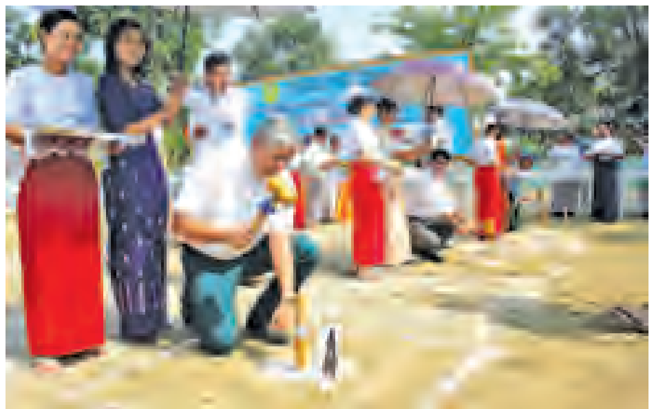
Director and Resident Representative of UNOPS Mr Sanjay Mathur drives a stake into the ground for construction of a sub-health centre in Kawton Village in Seikpyu Township, which is expected to be completed in December.—PHOTO: AYE MIN SOE
