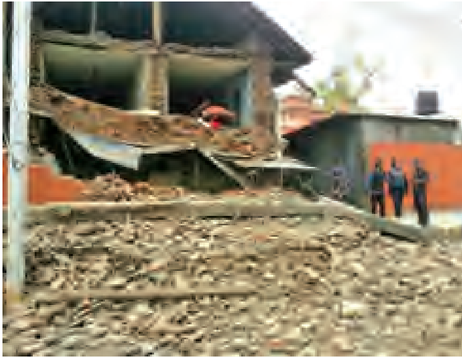
A collapsed building is seen in Nepal's capital Kathmandu on 25 April, 2015. An 8.1-magnitude earthquake struck Nepal, at 2:11 pm (Beijing Time) (0622 GMT) Saturday, China Earthquake Networks Center said.—XINHUA
