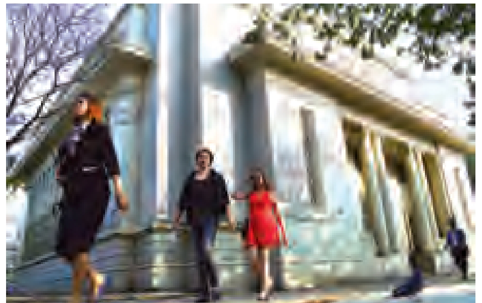
Pedestrians walk past a cultural heritage building where the Yangon Stock Exchange market will be established. —PHOTO: AYE MIN SOE
