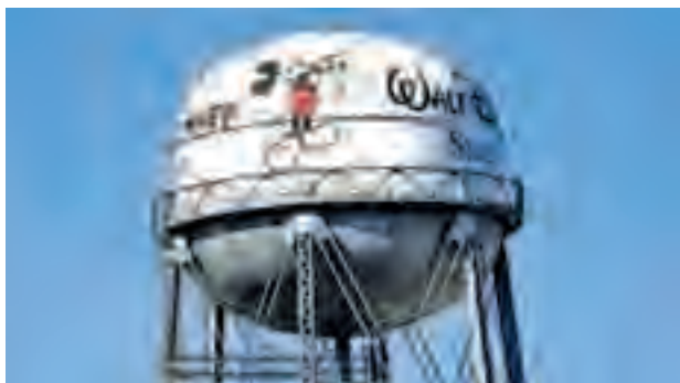
The water tank of The Walt Disney Co Studios is pictured in Burbank, California on 5 Feb, 2014.—REUTERS
