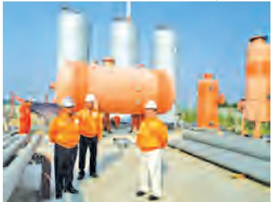
Deputy Minister for Energy U Aung Htoo visits Nitrogen Removal Unit in main natural gas control and distribution station in Ywama, Insein Township.—ENERGY
