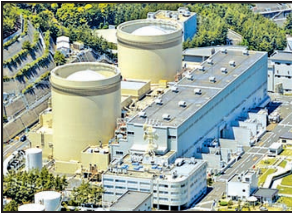
File photo taken May 2013 shows the Nos 1 and 2 reactors at the Mihama nuclear power station in the central Japan town of Mihama. Its operator Kansai Electric Power Co decided on 17 March, 2015, to decommission the two units, which have been operating for more than 40 years. — KYODO NEWS
