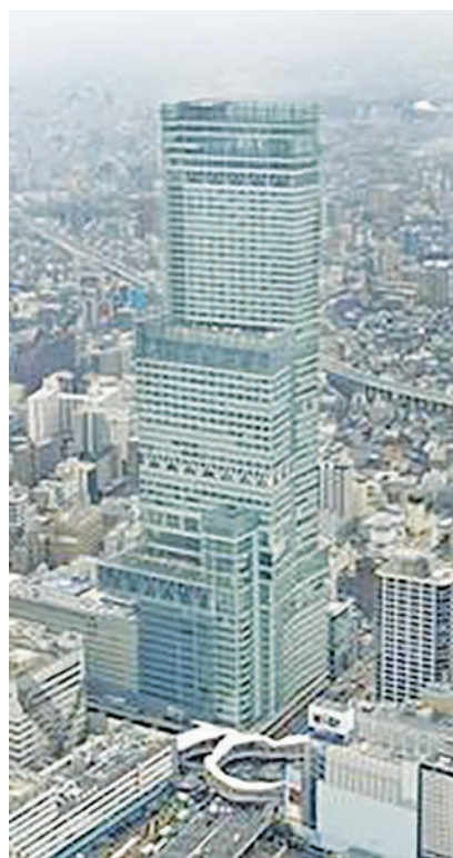
Photo taken from a Kyodo News helicopter on 7 March, 2015, shows Japan's tallest building Abeno Harukas in the western Japan city of Osaka. Its owner said the 300-metre-tall skyscraper drew a total of 42.73 million visitors in its initial year of operation, coming short of its first-year target of 47.4 million visitors. KYODO NEWS
