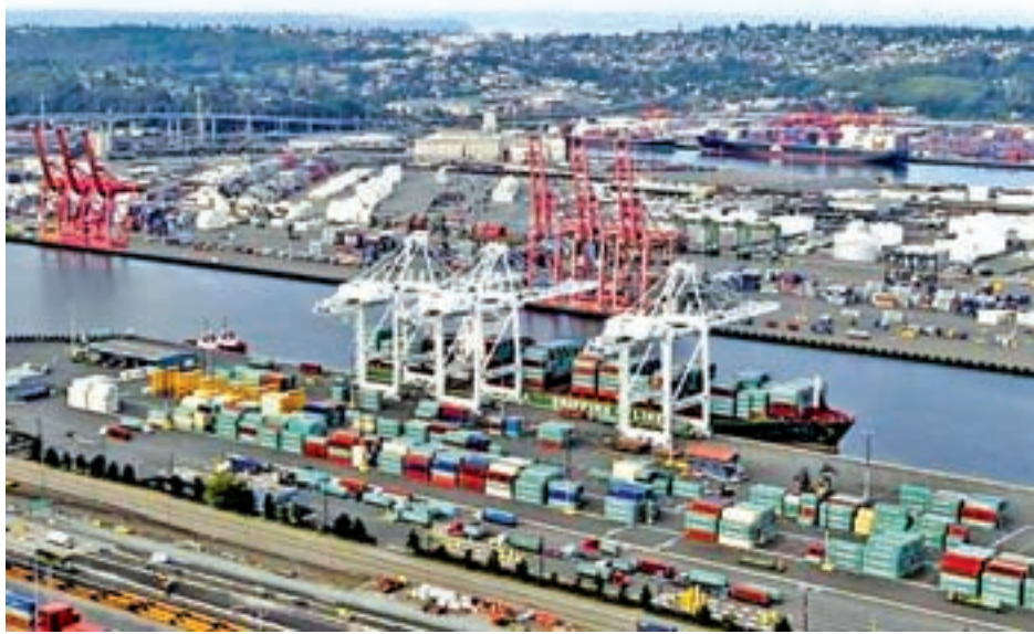
The shipping docks of the deepwater harbor of the Port of Seattle is seen on this aerial view photograph taken from a helicopter in Seattle, on 21 Aug, 2012.
