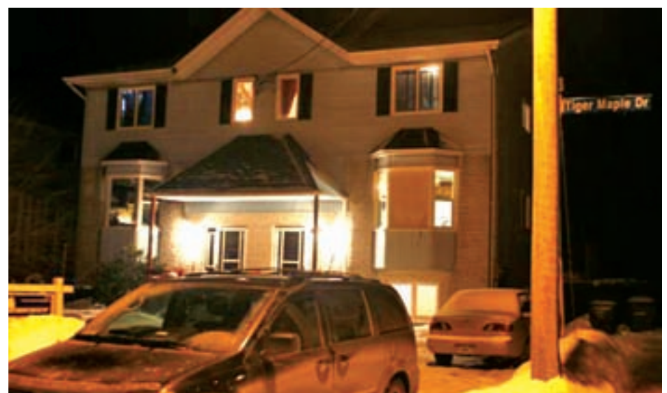
A duplex home where a 19-year-old man was found dead is shown in Timberlea, Nova Scotia, on 13 Feb, 2015. — REUTERS
