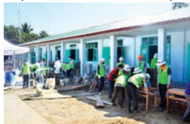
Korean students participate in construction of school building.
