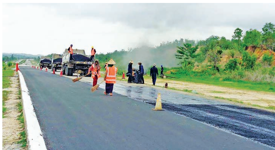
Skilled workers and engineers upgrading Yangon-Mandalay Expressway. CONSTRUCTION MINISTRY
