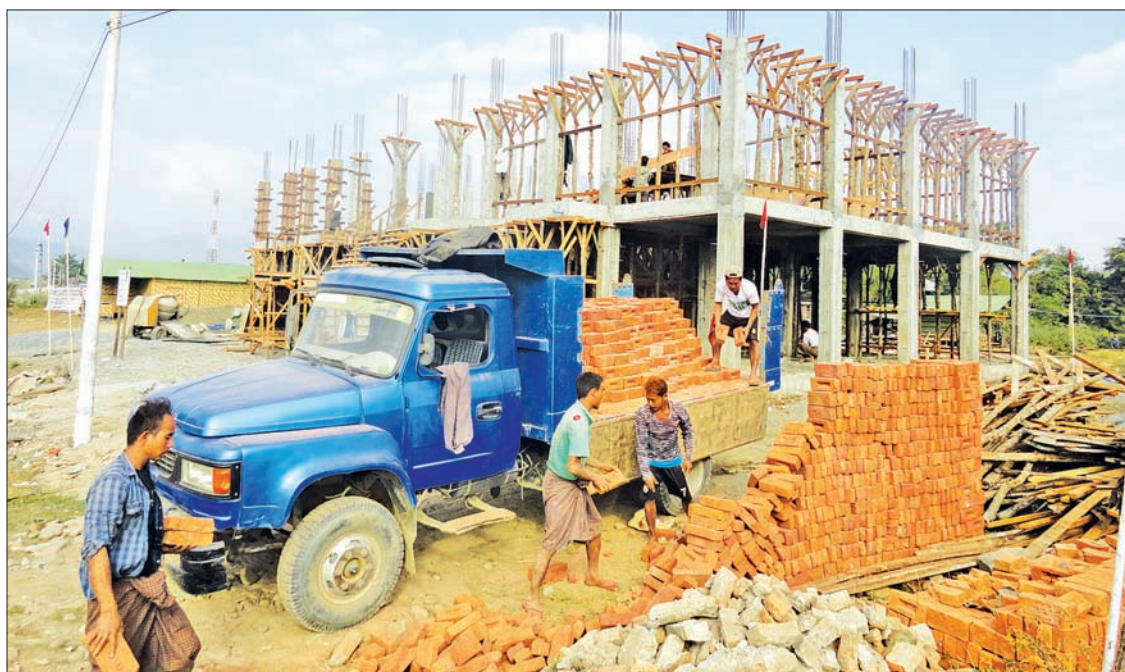
Traditional Medicine Hospital in Kalay is under construction. PHOTO: PON LUN-IPRD)
