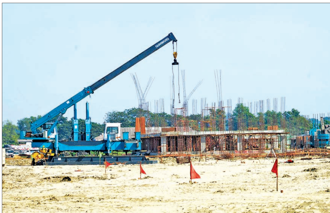
New vegetable and flower market under construction. PHOTO: ZAW MIN LAT
