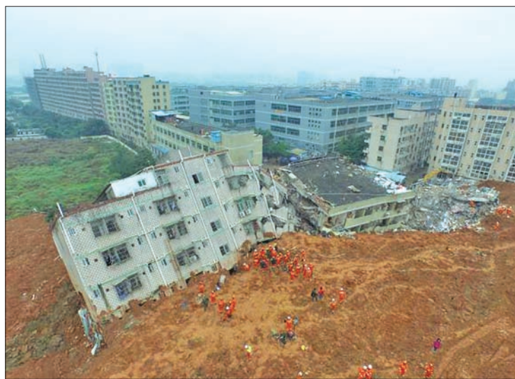
Firefighters search for landslide survivors among debris of destroyed buildings in Shenzhen, Guangdong province, on 21 December.
