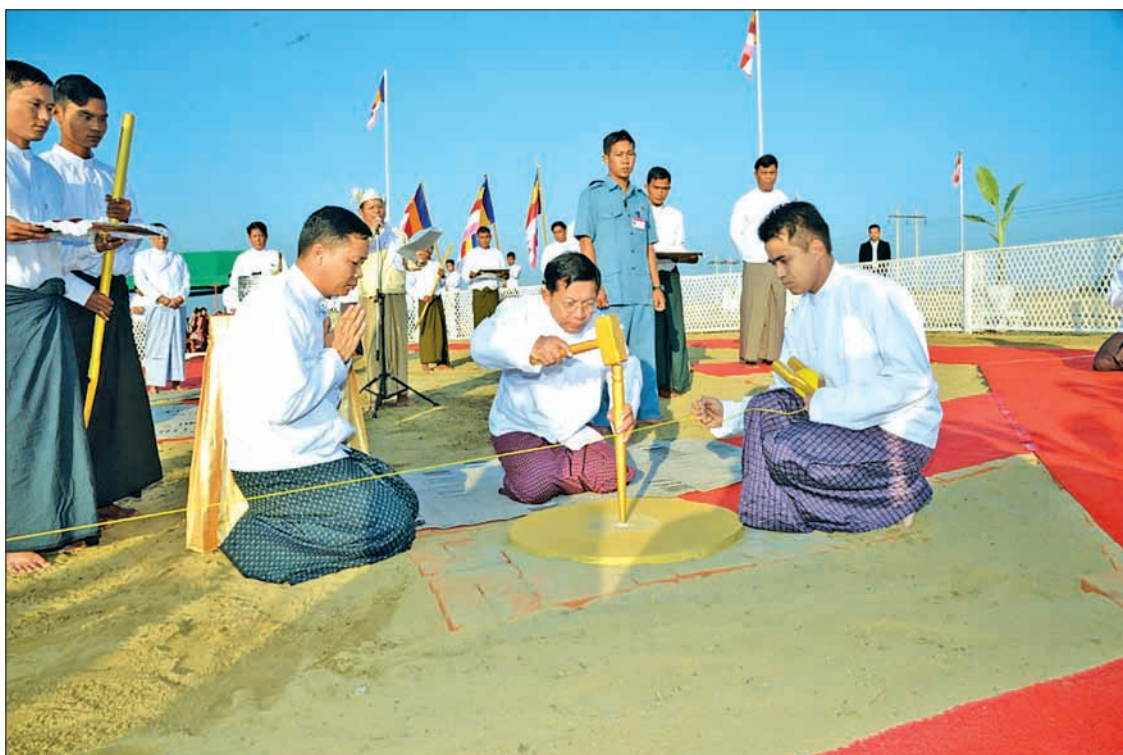
Senior General Min Aung Hlaing drives stake at a ground-breaking of home for aged for veterans. Photo: MNA
