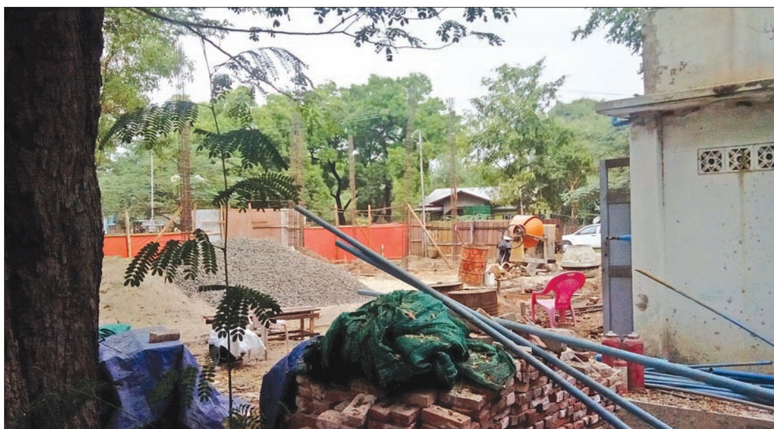
Refilling station is under construction in Mahlaing. PHOTO: STRINGER
