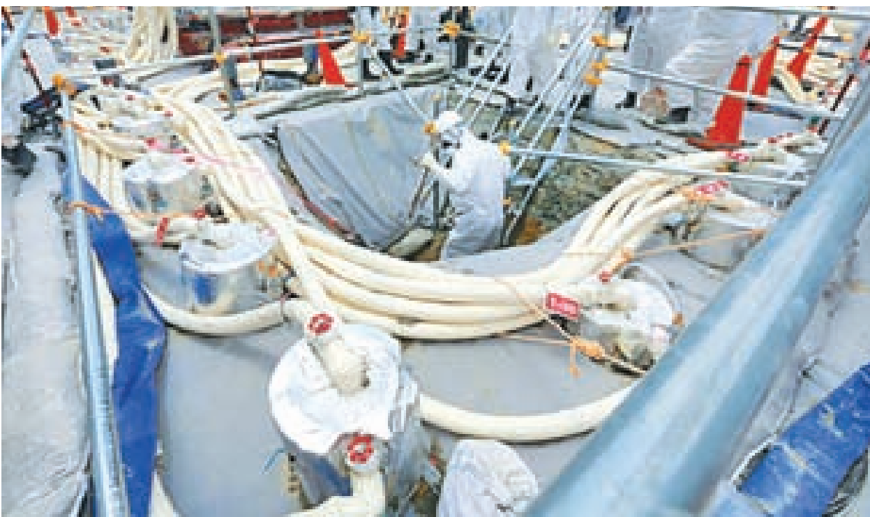
The government and general contractor Kajima Corp show an experiment to create underground walls of frozen soil to stop groundwater flowing into the reactor buildings at the crippled Fukushima Daiichi nuclear power plant in Fukushima Prefecture on 16 May, 2014. Cylindrical ducts to freeze soil are placed underground at 1-meter intervals.—KYODO NEWS
