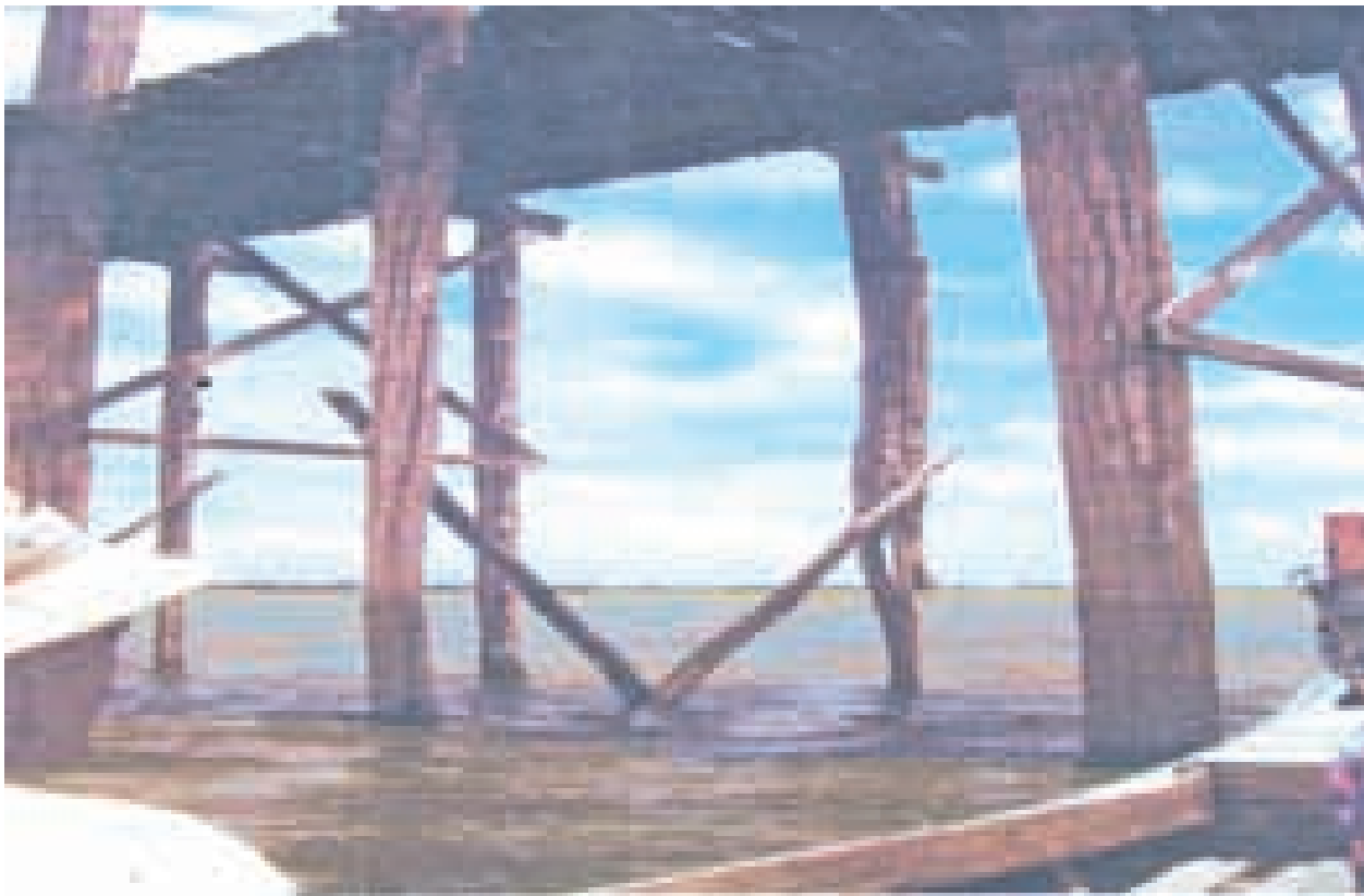
Photo shows decayed pillars of U Bein Bridge.—PHOTO MIN HTET AUNG
