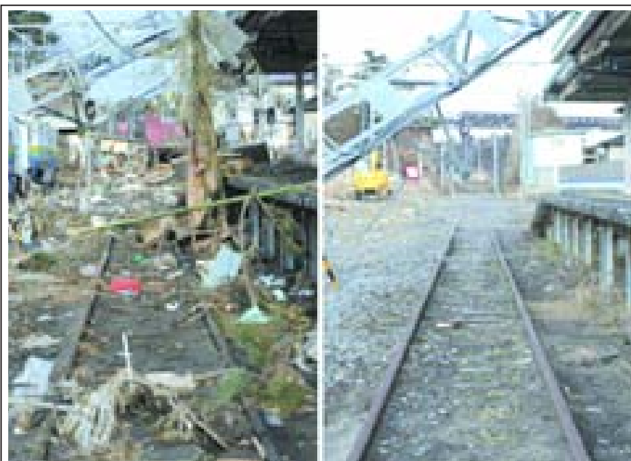
Photos show Nobiru Station on the JR Senseki Line in Higashimatsushima, Miyagi Prefecture, on 14 March, 2011 (L), three days after the Great East Japan Earthquake and tsunami, and on 3 March, 2014 (R). —KYODO NEWS
