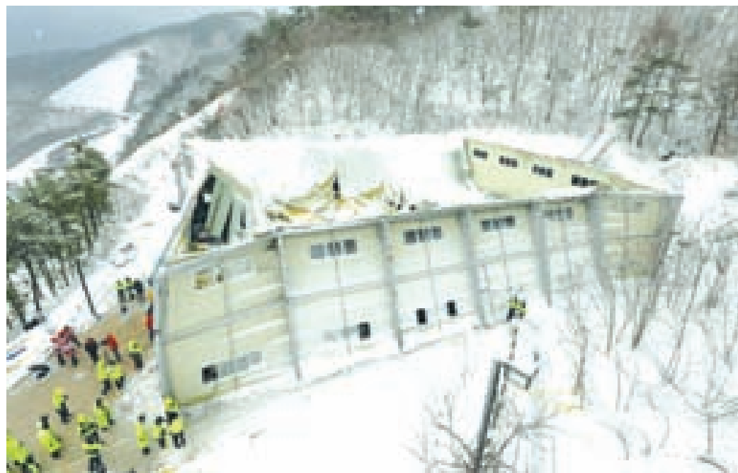
A 18 Feb, 2014, photo shows the roof of a gymnasium collapsed under the weight of snow in Gyeongju, South Korea. At least 10 people died and more than 100 were injured as more than 500 college students were having a welcoming party for freshmen in the building when the roof collapsed on 17 Feb. KYODO NEWS
