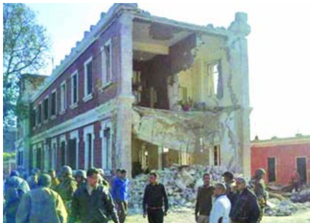
People and army personnel stand around a damaged building after an explosion in Egypt's Nile Delta town of Anshas, about 100 km (65 miles) northeast of Cairo, on 29 Dec, 2013.—REUTERS
