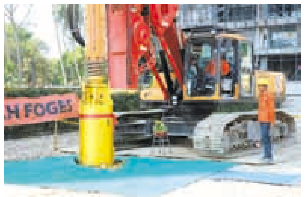
Stake-driving ceremony of Shangrila Lakeside Hotel construction in progress.
