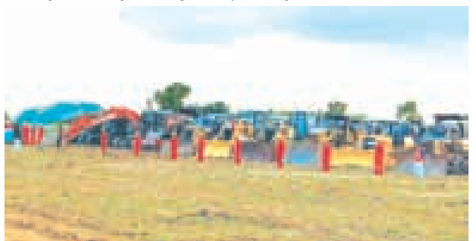
Photo shows machinery being used in Thilawa Special Economic Zone.
