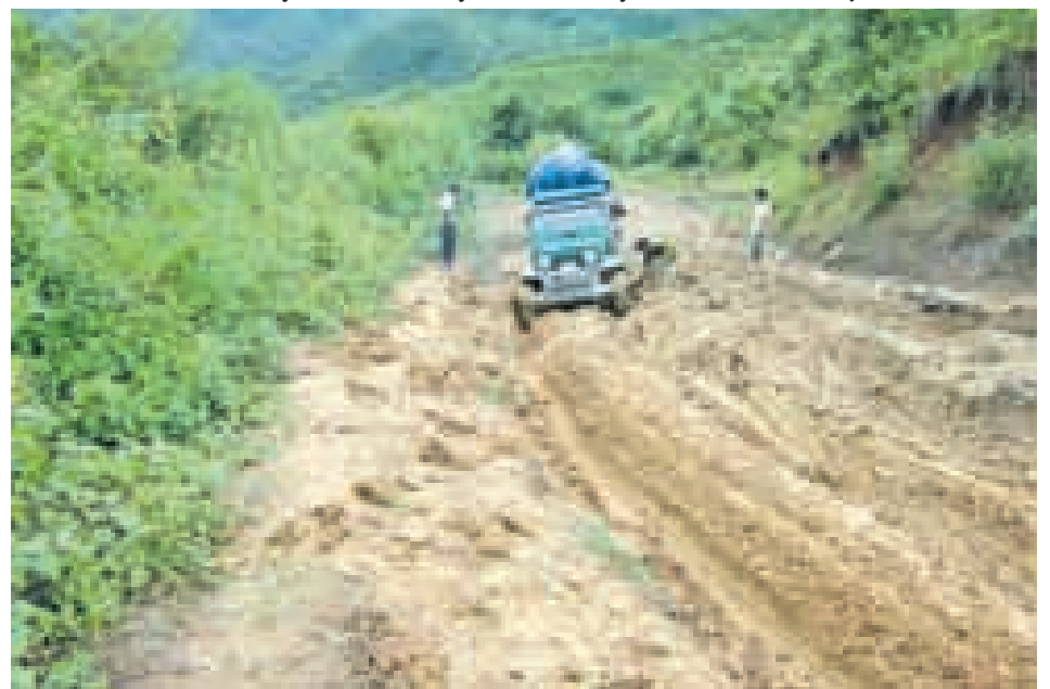
Photo shows poor transport facility on Kalewa-Yargyi road section.
