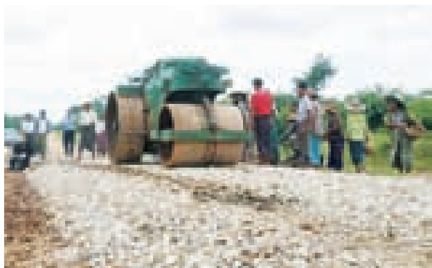
Earthen road being upgraded with gravel linking Kanni and Magyisu villages in Meiktila Township.
