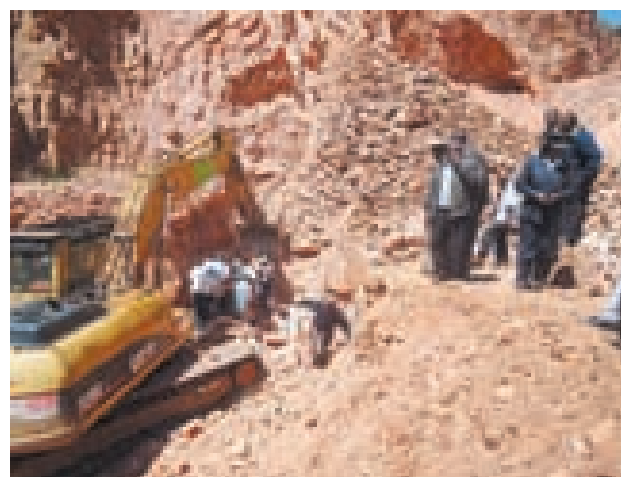
Rescuers work at the quarry collapse site in Bomet county, southwest of Kenya, on 25 Oct, 2013.—XINHUA
