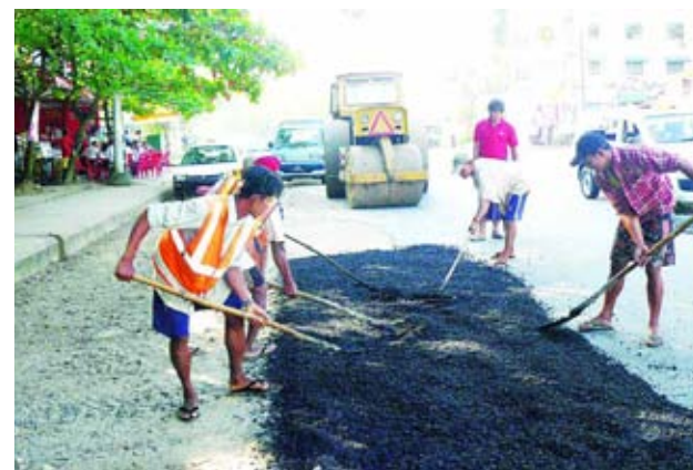
Yangon City Development Committee is striving for ensuring convenient travelling and smooth transportation of the people. With the aim of keeping traffic accidents and congestions from away, Engineer in-charge U Cho Win and party of Road and Bridge Department of Ahlon Township Development Affairs Committee repairing damaged road sections on Lower Kyimindine Road in front of Ahlon Myoma Police Station on 24 October morning.
